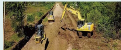
A hydraulic excavator operating for infrastructure development in Cambodia
