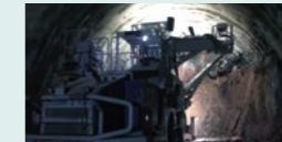
Drill Jumbo in operation for mountain tunnel construction
