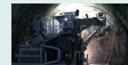
Drill Jumbo in operation for mountain tunnel construction
