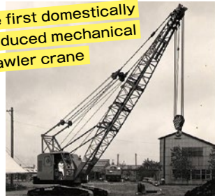
Ishikawajima Harima Heavy Industries (currently Kato Works) 330 sprawler crawler crane (1952) This mechanical crane was manufactured by Ishikawajima Harima Heavy Industries, a company set up based on a technological tie-up between Ishikawajima-Harima Heavy Industries and Calling (US).
