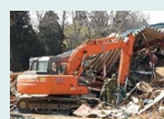
"ZX120" cleaning up debris
